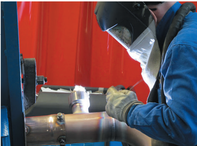
Welding CuNi piping spools
